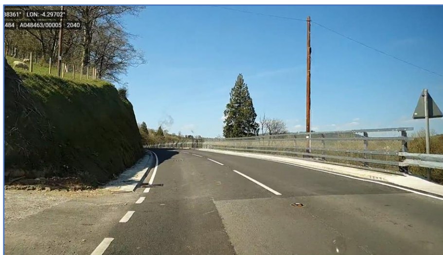
A484 Pante Retaining Wall
